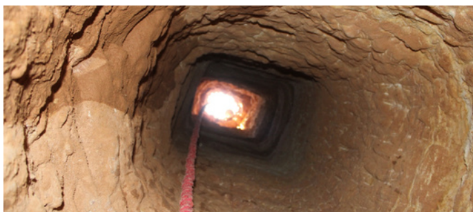
Aeration well, Adrar, undergoing community work to maintain the foggara (Image: J.I. Robles, 2025)
